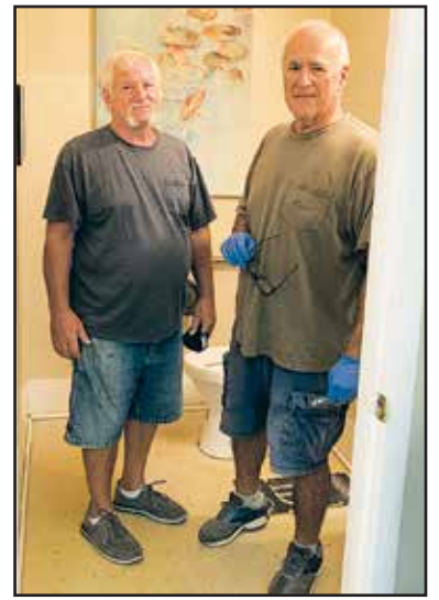
Doug Link and Joe Farina replaced our client's restroom floor. Joe built a new vanity.
